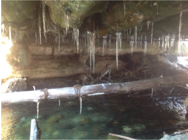
Right Bank Abutment when facing downstream
