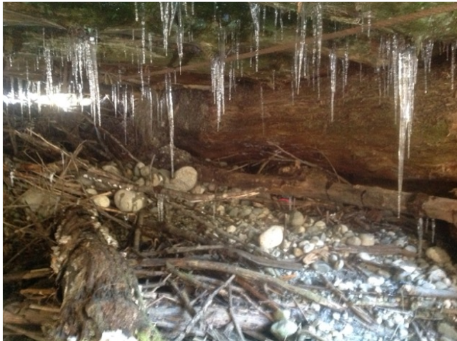
Left Bank Abutment when facing downstream
